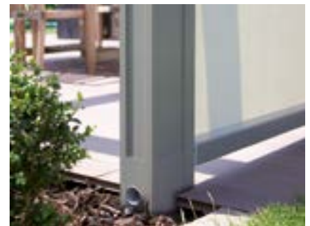
Integrated water drainage
