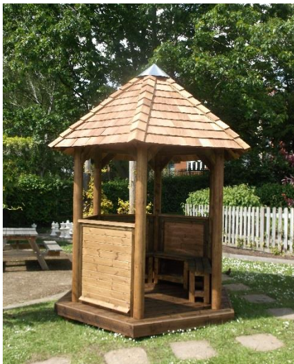
Completed Reading Hut
