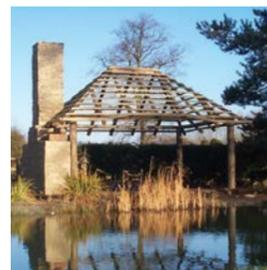
At the heart of every Lapa is an extremely strong timber frame which, due to the design, does not require sections of raftering to provide strength. In our view these limit access and potential uses. The frame will be constructed
