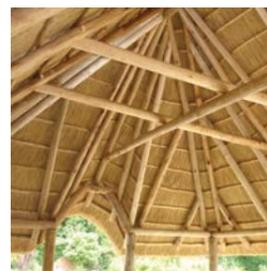
To ensure the strength of these structures, Lapas are built using a 100% timber frame. Not only does this give a natural product, but it looks fantastic and accurately re-creates structures found in South Africa. We would not consider using
